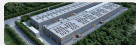
Shanwei Luhe Facility 62360m 2
