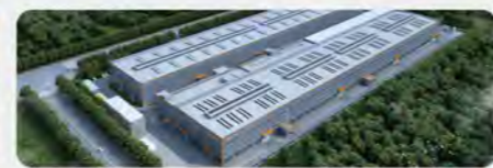
Shanwei Luhe Facility — 62360m 2
