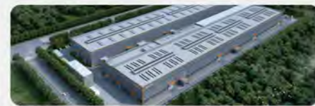
Shanwei Luhe Facility 62360m 2
