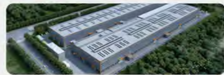
Shanwei Luhe Facility 62360m 2
