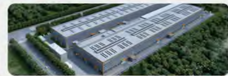
Shanwei Luhe Facility 62360m 2
