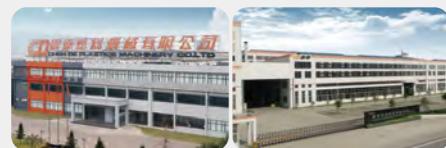
Foshan Shunde - Two Facilities 150000m 2
