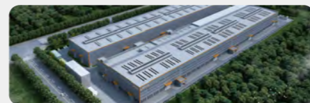
Shanwei Luhe Facility 62360m 2
