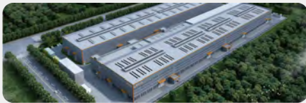
Shanwei Luhe Facility 62360m 2
