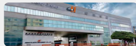
Taiwan Taoyuan Facility 30000m 2
