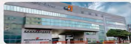
Taiwan Taoyuan Facility 30000m 2
