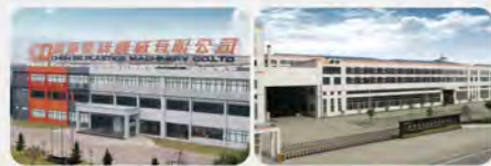
Foshan Shunde - Two Facilities 150000m 2
