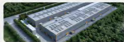
Shanwei Luhe Facility — 62360m 2
