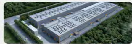
Shanwei Luhe Facility 62360m 2
